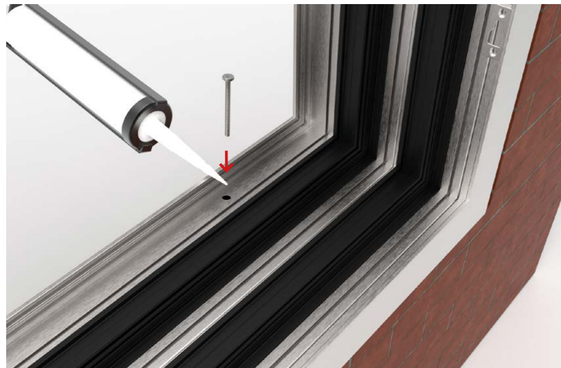
4 Insert suitable sealant to fixing hole, then screw preferred fixing in place. Repeat process along the bottom track, ensuring fixings are within 600 mm intervals.
